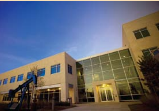
PTRC building located in Regina (Photo courtesy of Petroleum Technology Research Centre)
